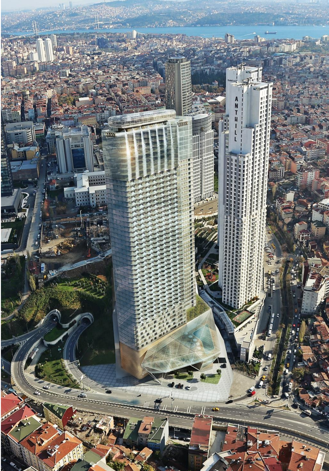
150.000m 2 , SİNPAŞ GYO BOMONTİ QUEEN CENTRAL PARK 55 STORY REINFORCED CONCRETE RESIDENCE
